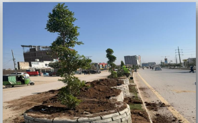
Planters Work at Ring Road
