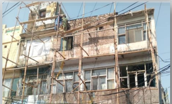
Renovation of Super Market Phase-I - Peshawar
