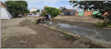
Walkway Under Construction
