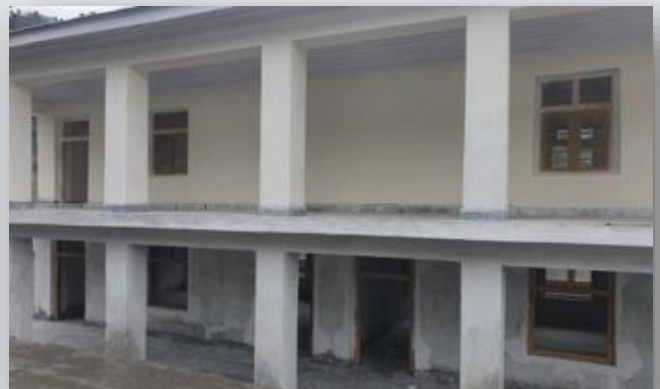
Construction of classrooms at Chitral Lower
