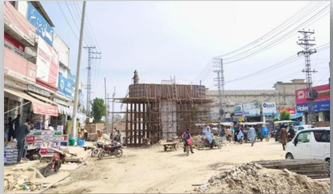
Flyover construction – DI Khan
