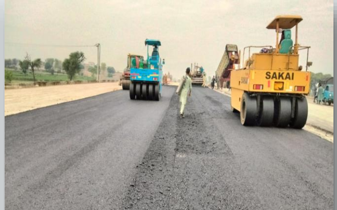
Northern Section Ring Road - Peshawar
