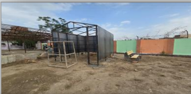
Tuck-Shop Under Construction
