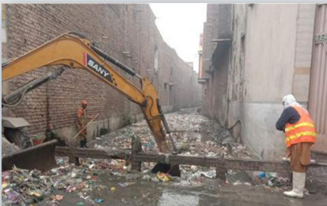
Sewers desilted in Peshawar
